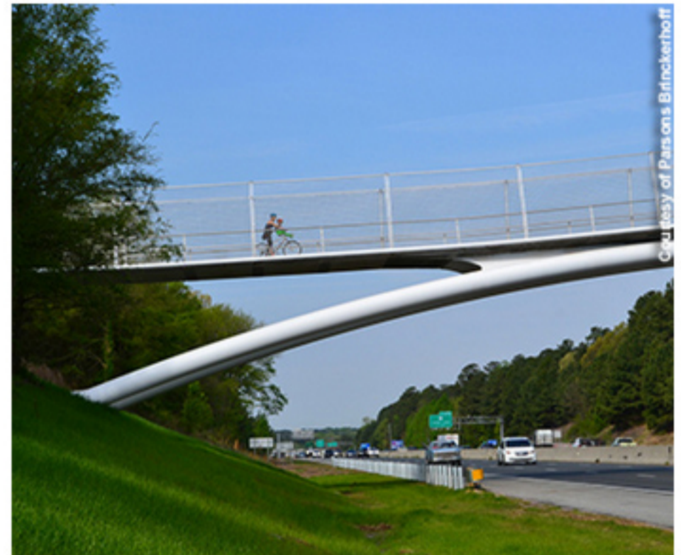
The $5.5-million American Tobacco Trail Bridge—the largest hybrid stressed ribbon bridge in the United States—will be officially completed within the next few weeks. It conducts a bicycle and pedestrian pathway over Interstate 40 in Durham, North Carolina. Courtesy of Parsons Brinckerhoff
