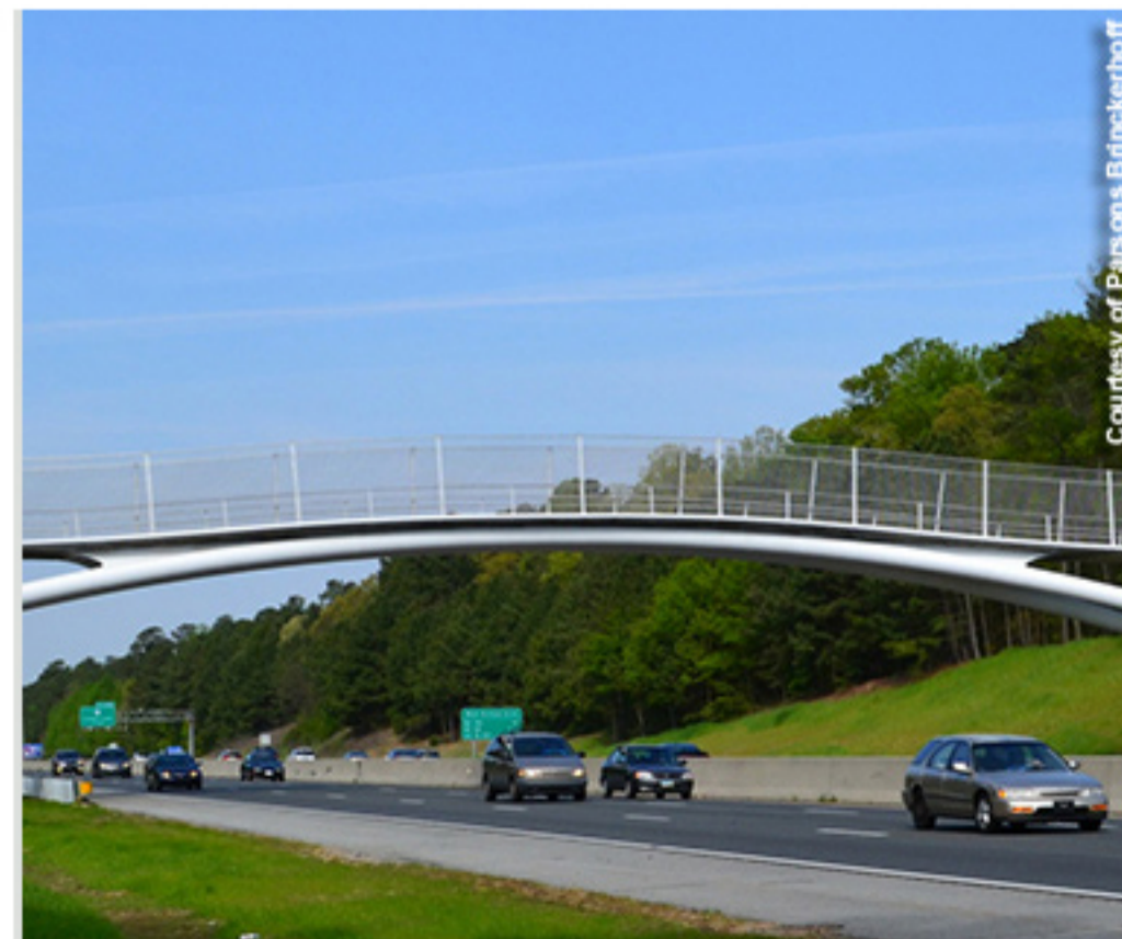
The self-anchored bridge spans 210 ft between its arch supports. It combines a 268 ft long, 9 in. thick concrete stressed ribbon deck with two 30 in. diameter curved steel arch ribs. Courtesy of Parsons Brinckerhoff
